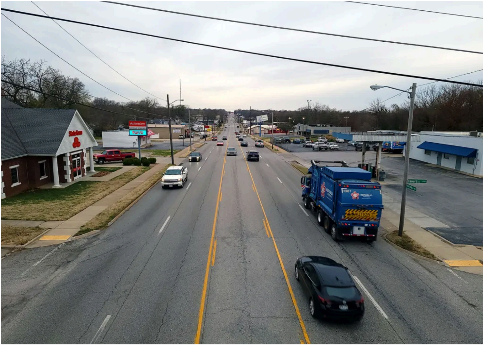
Kearney Street, as seen looking west toward Grant Avenue, will serve as a detour route amid upcoming construction in Interstate 44. (Photo by Shannon Cay Bowers)
