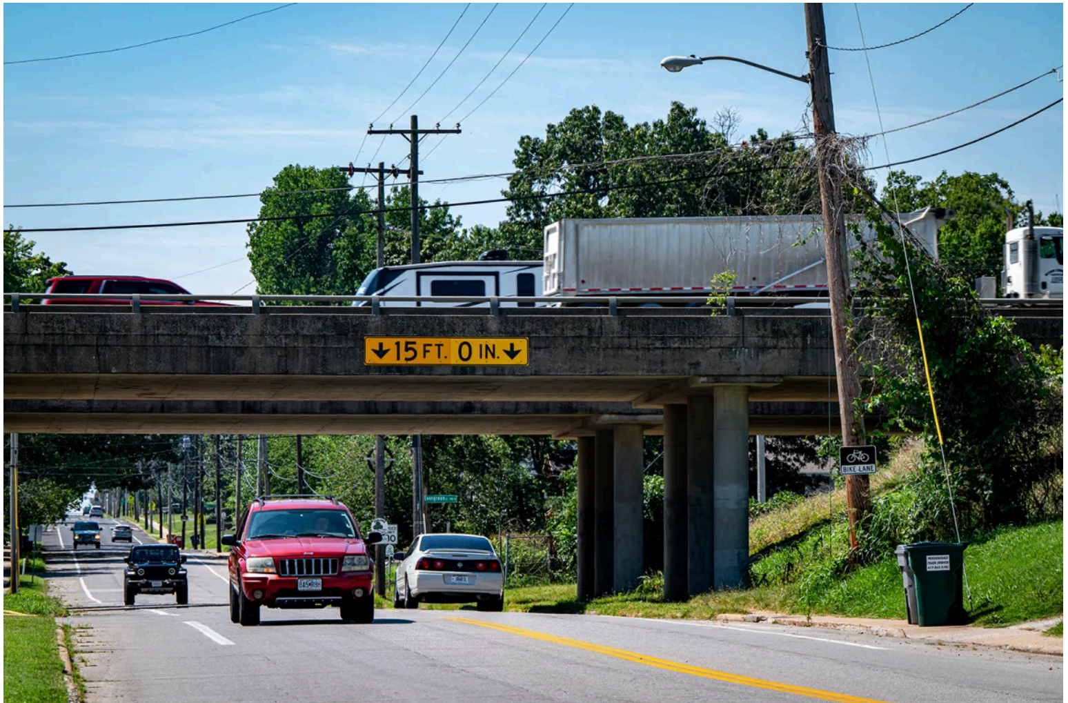
Traffic heading north on Grant Avenue passing under the overpass carrying Interstate 44. (Photo by Jym Wilson)
